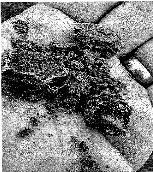
Photo 3: A small asphalt chunk within the top 5".
