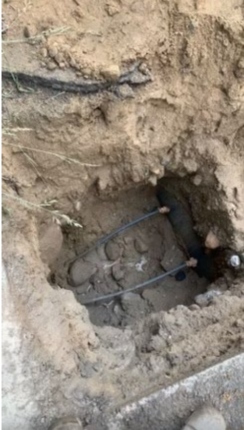
1 Plastic Water Service prior to replacement
