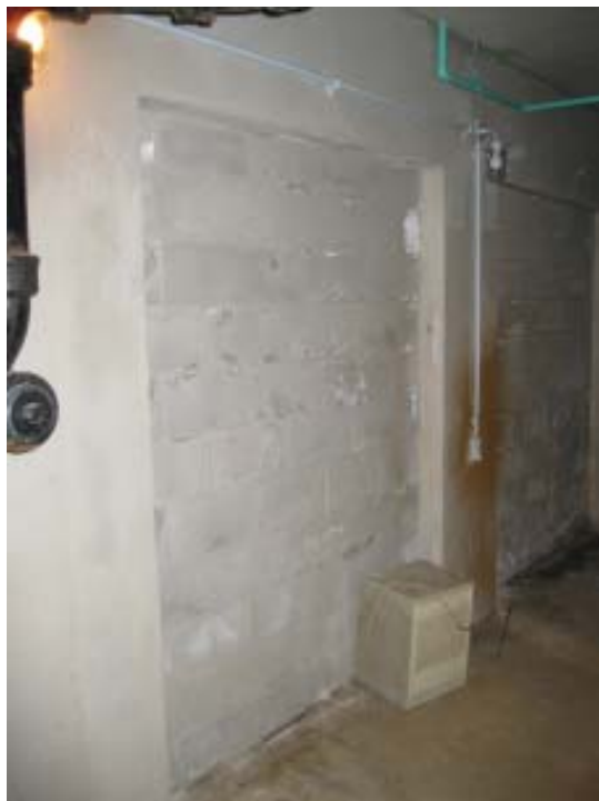
Photo 9 - Masonry knock-out wall in basement level,
