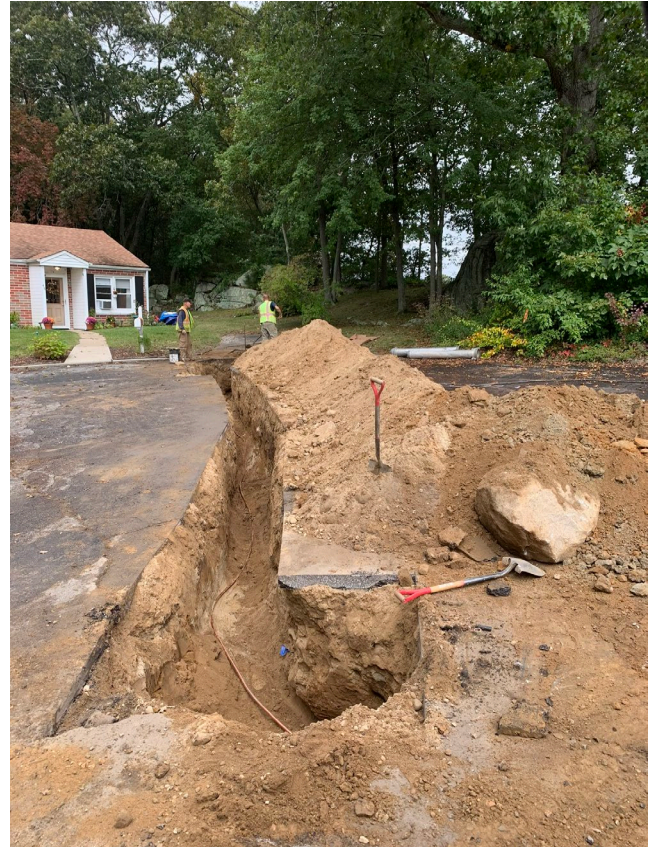
2 Plastic Water Service Replaced with Copper Line
