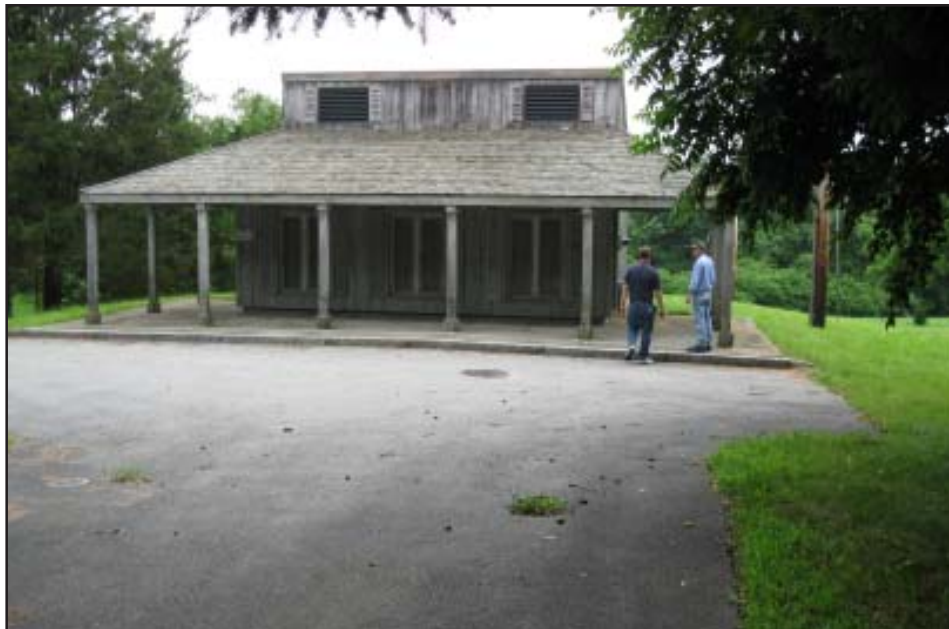
Photo 1 - Front of building.
