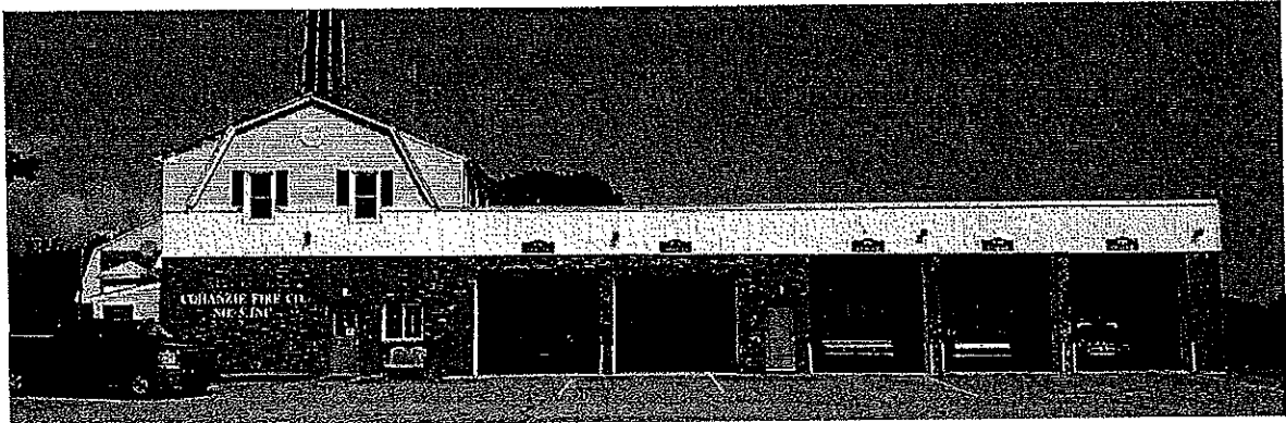
Figure 2- Cohanzie Fire Station
