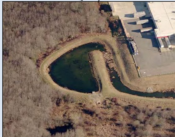
Water Quality Basin
