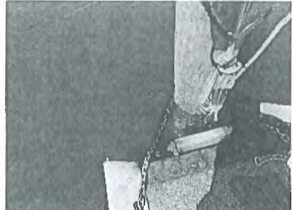
Floating Precast Dock Finger & Timber Pile
