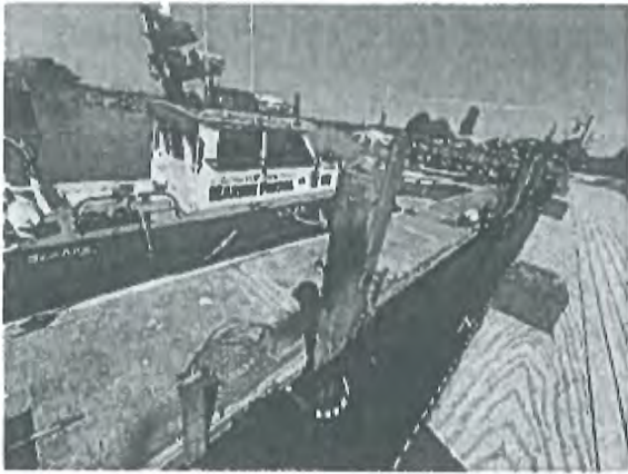
Looking Northwest – Floating Dock & Timber Piles
