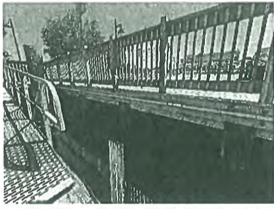
Looking Northeast – Trex Deck Support Structure Adjacent to the Dock System
