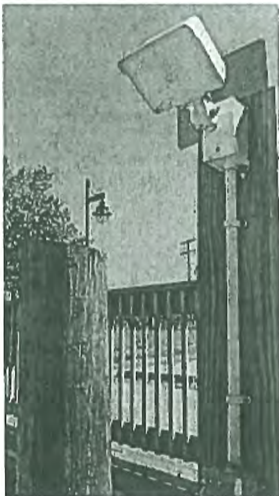
Pole mounted area light fixture
