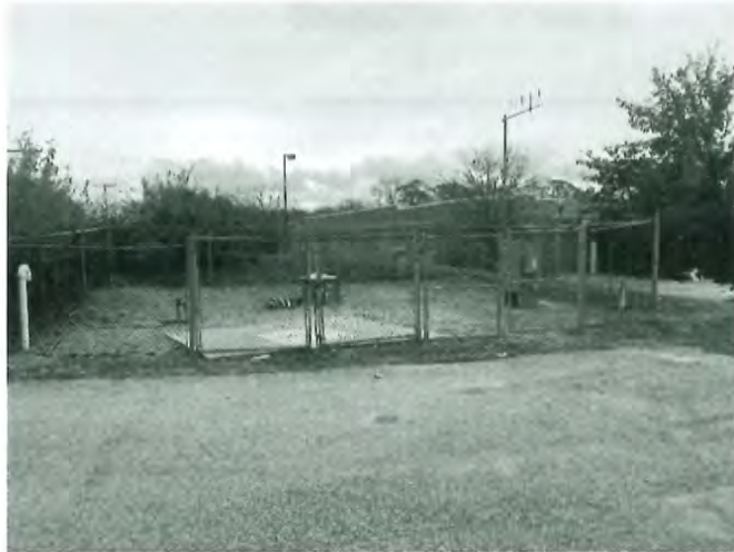
Route 85 Wastewater Pump Station
