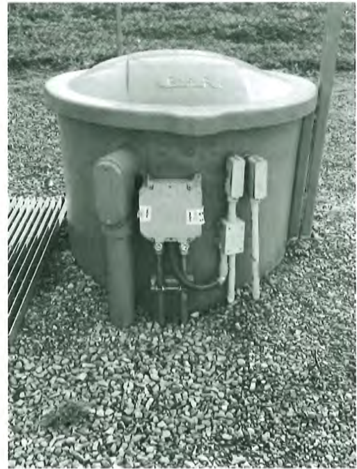
Route 85 Wastewater Pumping Station Manway
