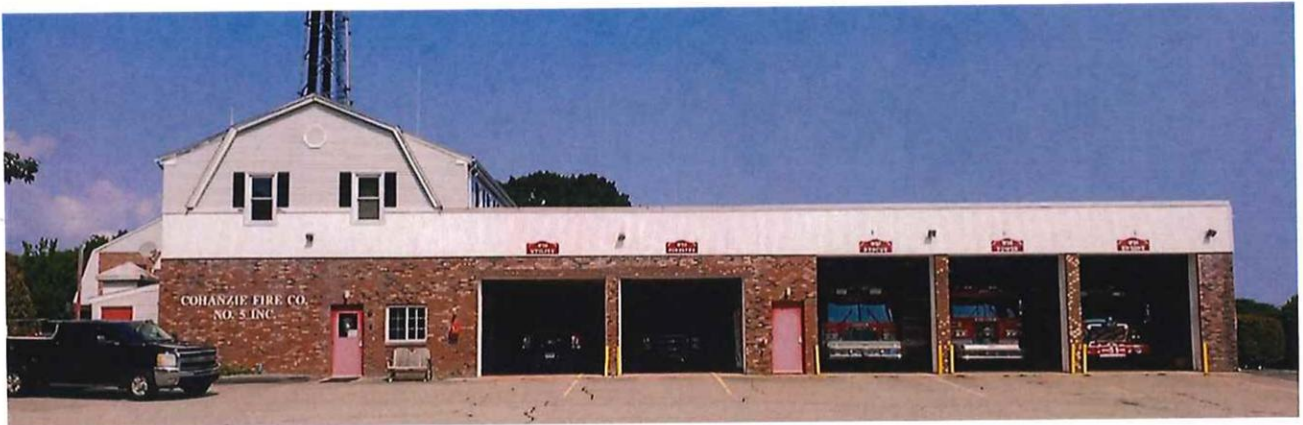
Figure 2- Cohanzie Fire Station
