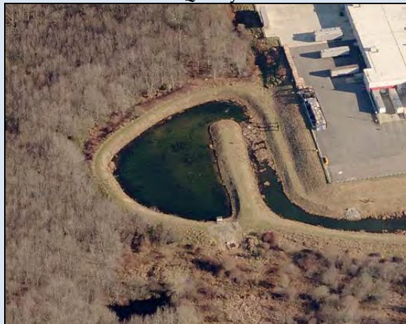
Water Quality Basin
