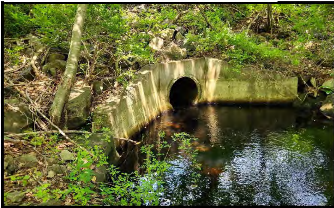
Picture 3 - Detention Basin Discharge Culvert
