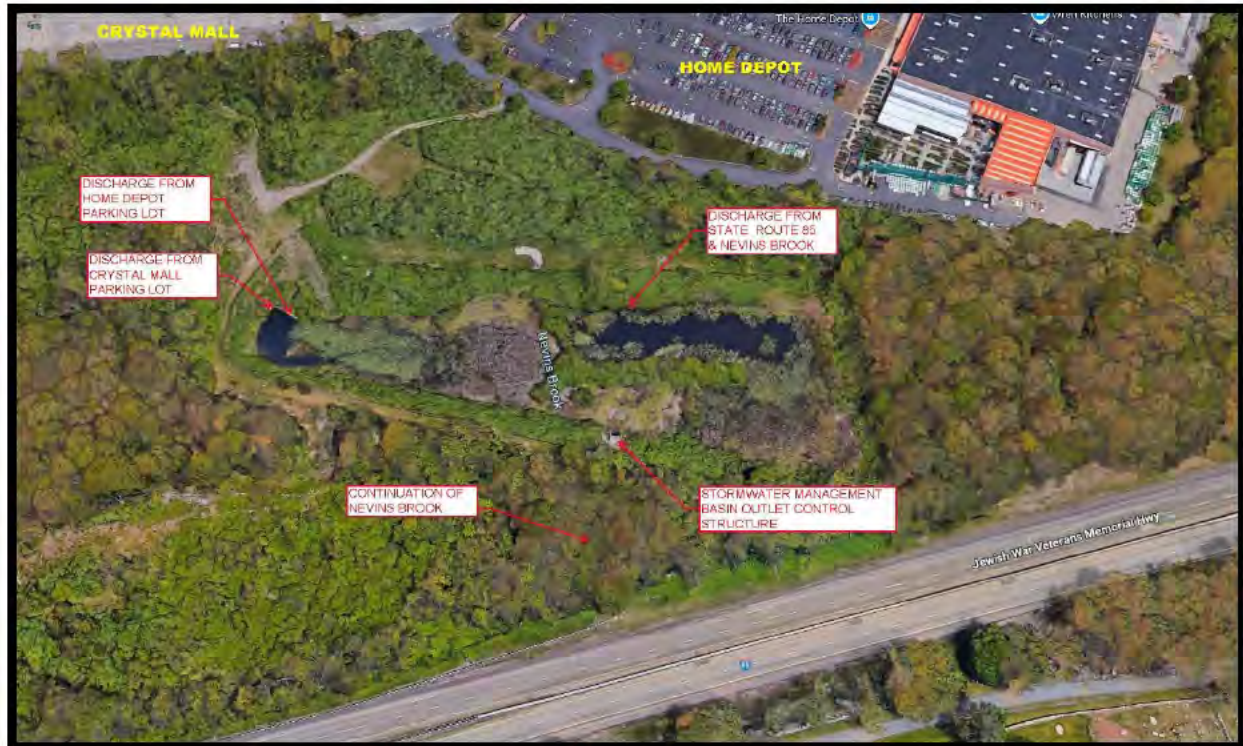
Picture 1 - Aerial View of the Existing Stormwater Management Basin (A.K.A. Trading Cove Pond)
