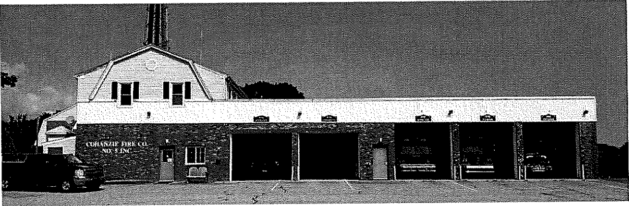
Figure 2- Cohanzie Fire Station
