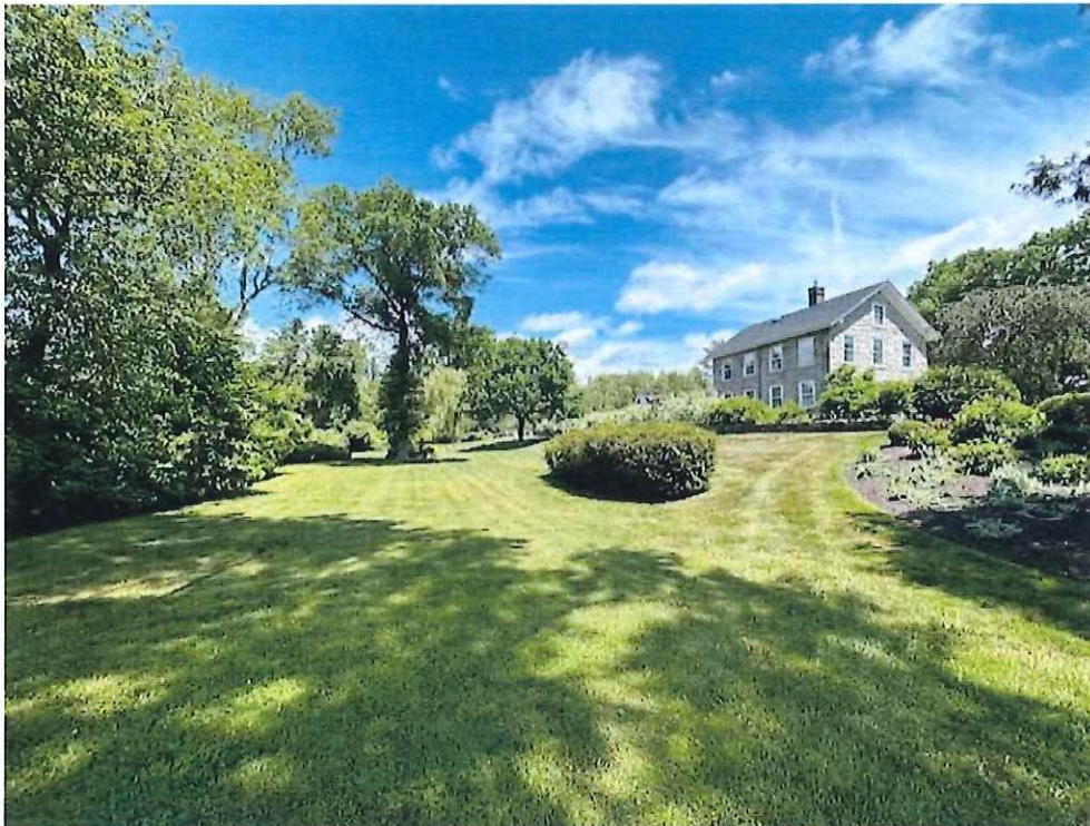
Photo 4: Example of the general conditions of grounds that surround the historic Granite House.
