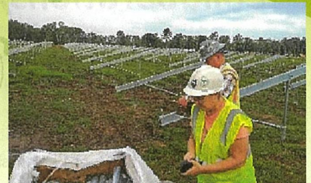
ECCD staff inspect erosion & sediment controls at a solar site.
