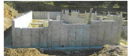
Construction commenced a multi-phase nutrient management initiative, including construction of a free-stall barn with manure storage..
