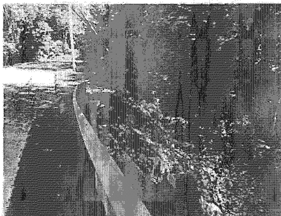
Picture 2 – Repaired Embankment at the Northeast Corner
