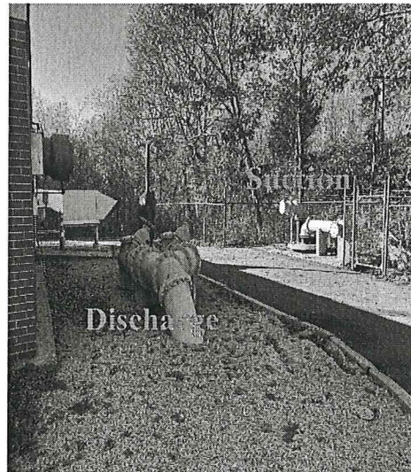
Emergency By-Pass Discharge Piping
