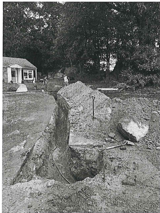
Plastic Water Service replaced with copper line
