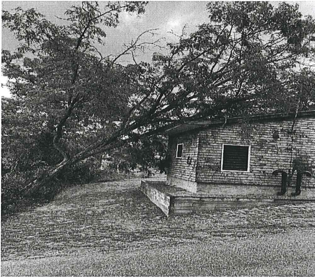
Niantic River Road Station Before New Roof
