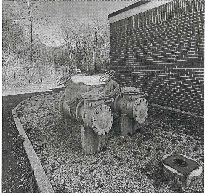
Emergency By-Pass Discharge Piping
