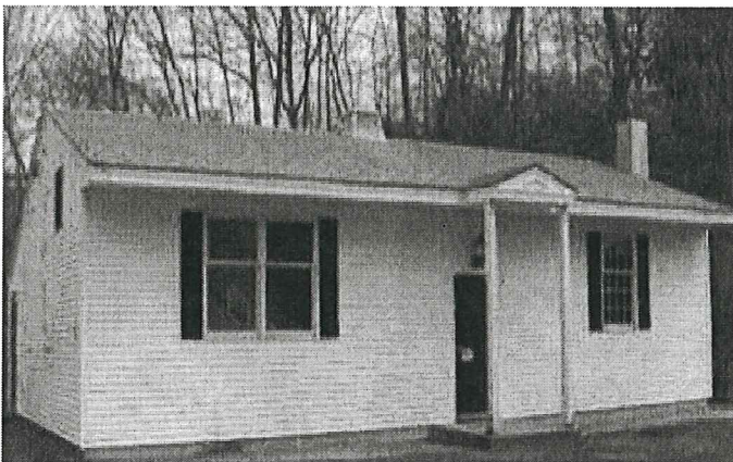
Bolles Court Station Before
