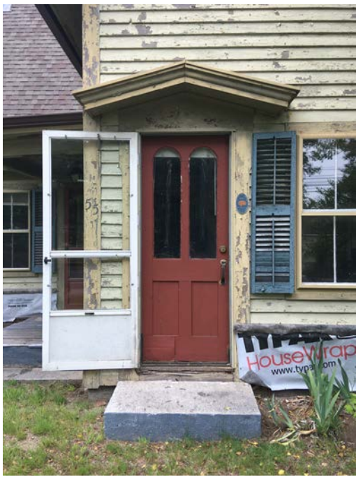
FRONT DOOR, SOUTH ELEVATION
