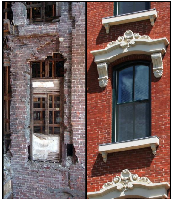
Wauregan Hotel (c. 1850) – Building Envelope Repair and Structural Stabilization (Photo © Pietro Camardella)
