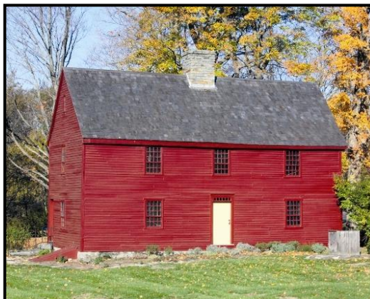
Hurd House Museum (c. 1682) –In-Place Structural Repairs to Sills and Upper Floor End Girts
