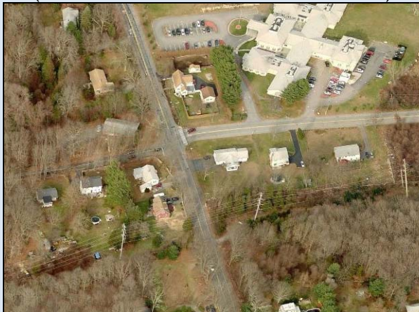
Collector Road (Vauxhall Street Extension at Greentree Drive)
