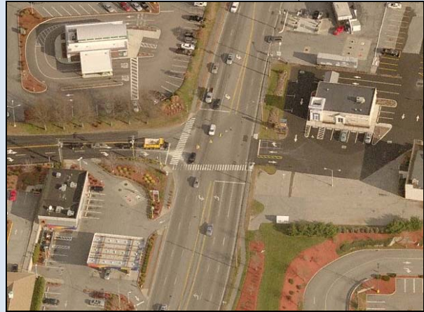
Arterial Road (Route 1 at Clark Lane)
