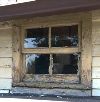
Window #208 above low roof
