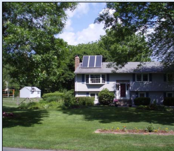
Residential Solar Collector
