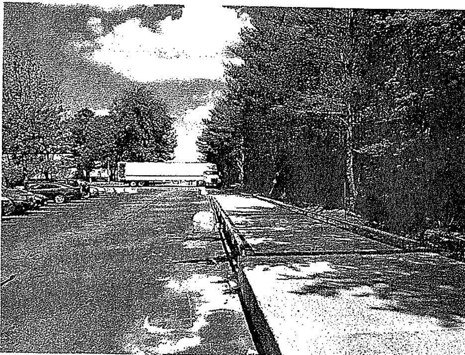
Example of pre-cast deck scale in existing foundation. Scale replaced fatigued platform and was operational in under 2 days.
