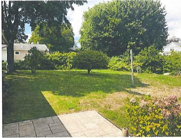
Photo scanning the overgrowth covering about a 100' section of the channel on 19 Nichols Lane
