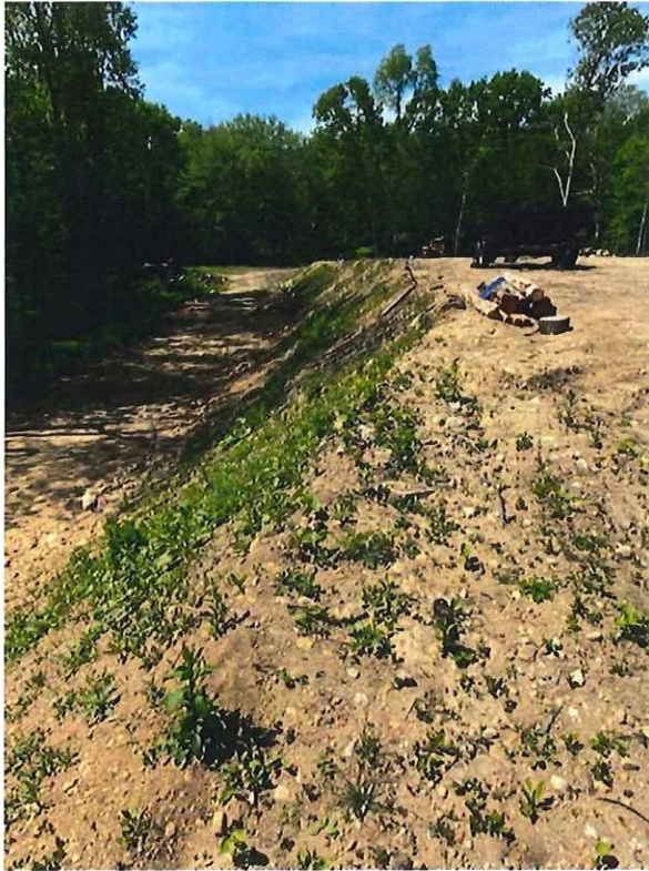
Clearing of vegetation and grading of approximately 200 linear feet of a hillslope
