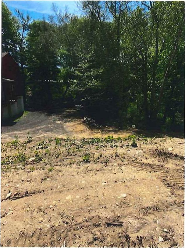
Deposition of earthen fill and asphalt millings west and south of the barn outbuilding
