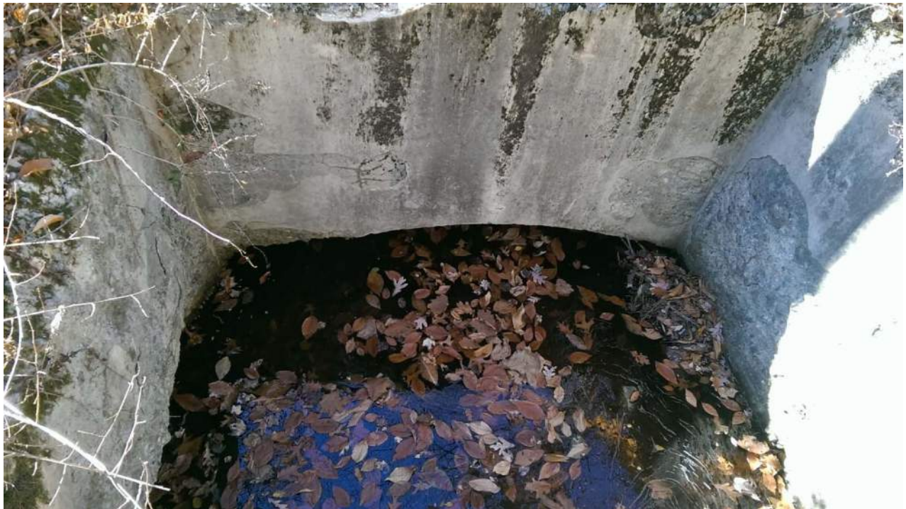
PHOTO 10: View of watercourse outlet from bridge.
