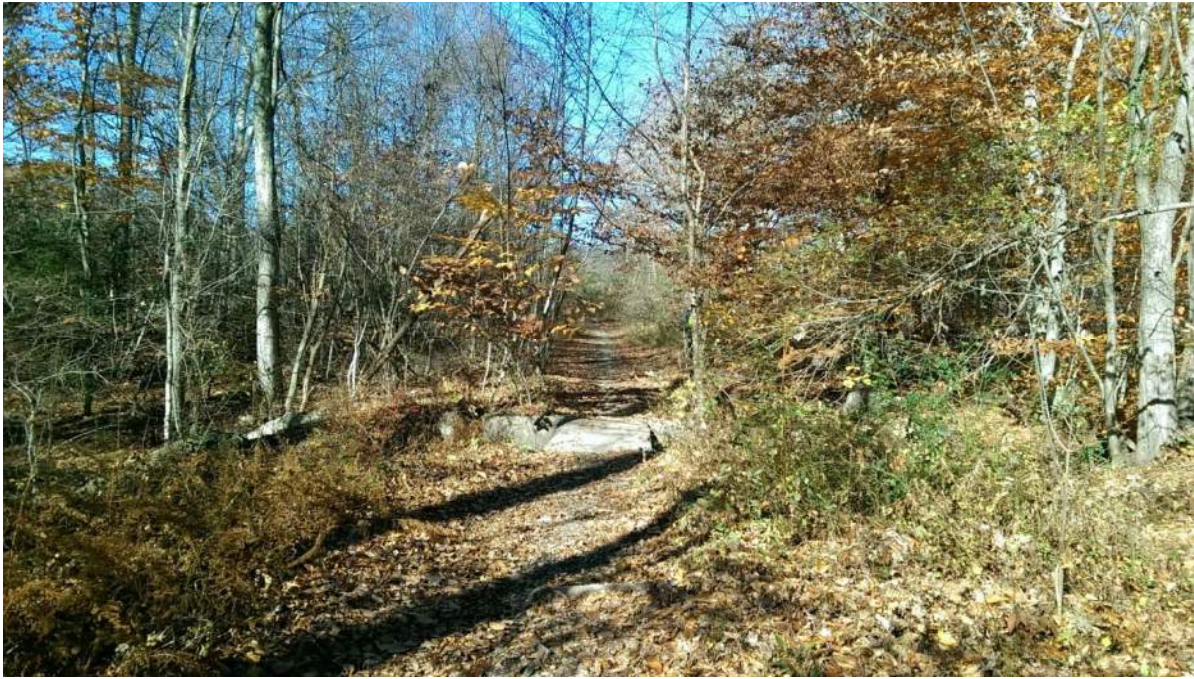
PHOTO 9: View of dirt access road and bridge over watercourse 1.
