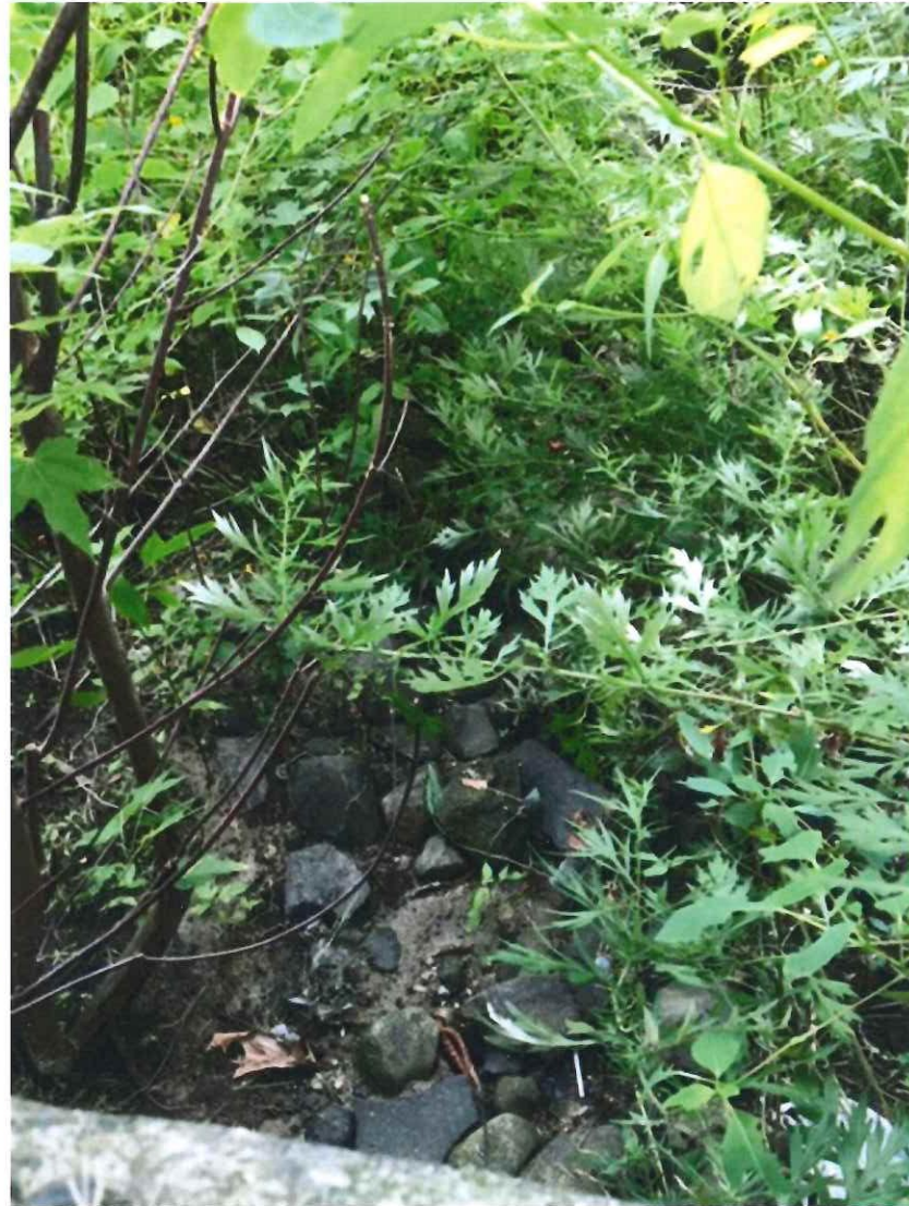
View of outfall area from headwall Fifth Avenue
