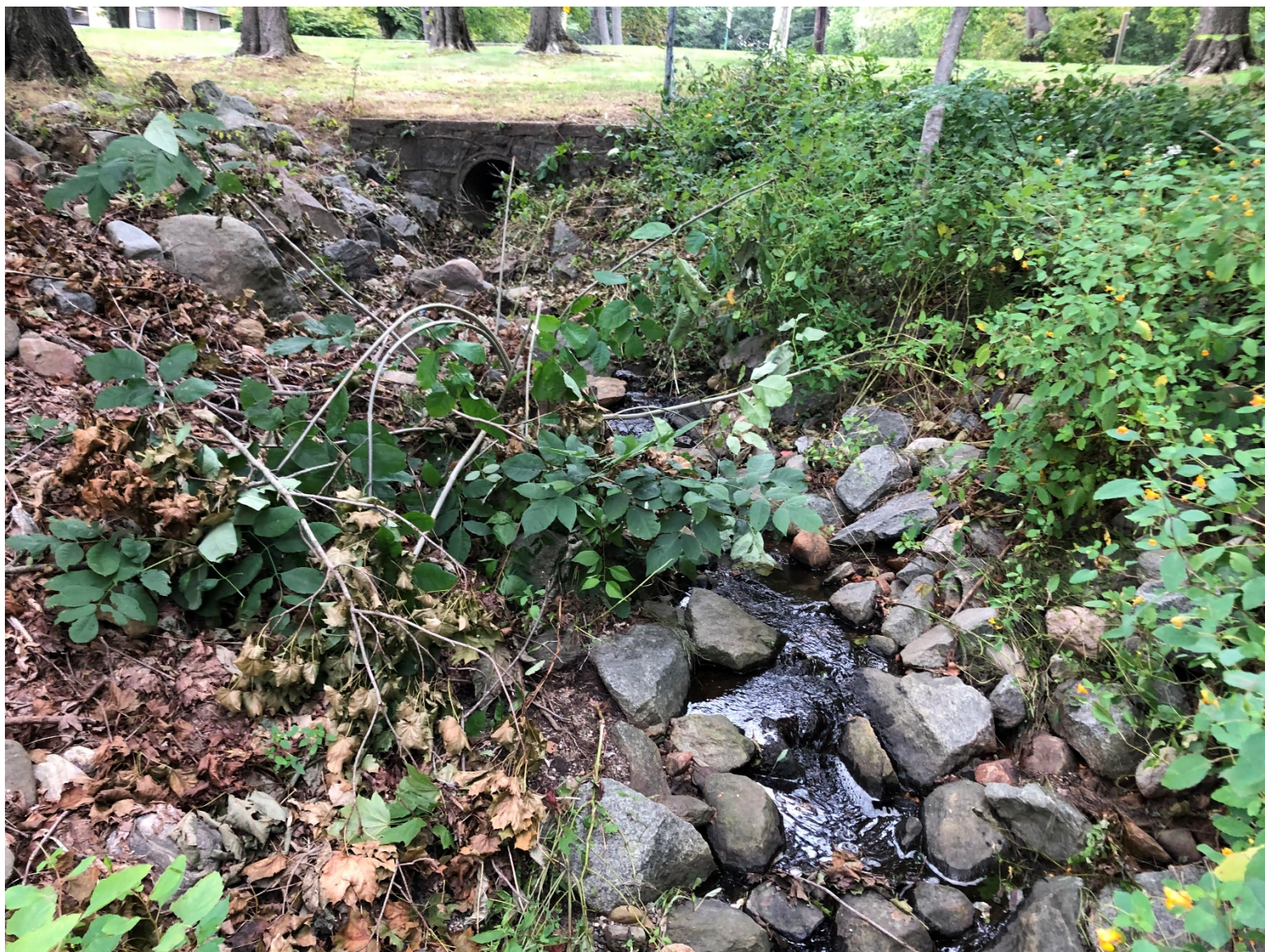
Rip-rap at pipe outfall September 8, 2021
