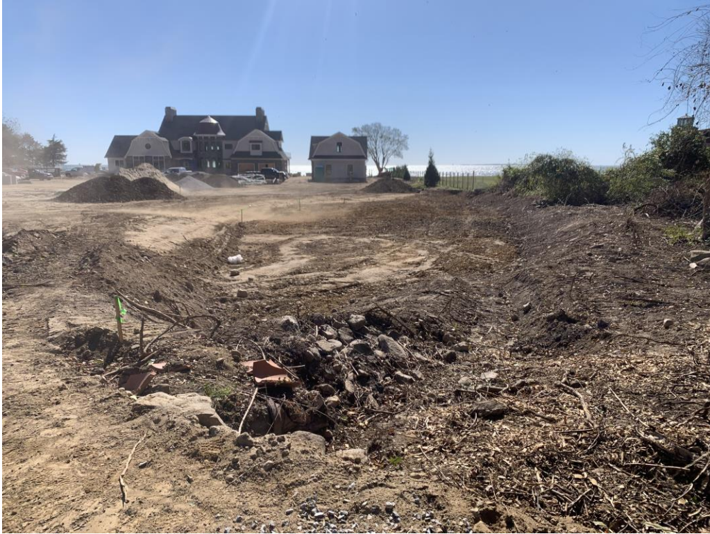
Photo 2: October 8, 2021 – Rough Grading Inspection
