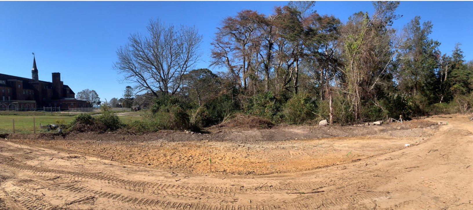
Photo 1: October 8, 2020 – Rough Grading Inspection
