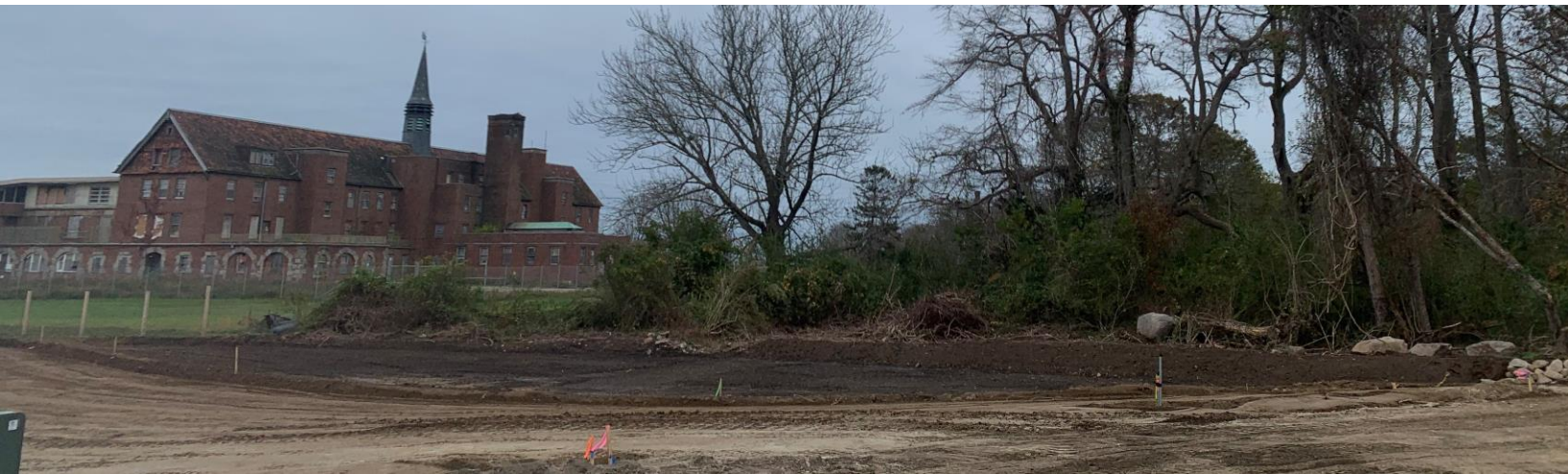
Photo 4: October 20, 2020, Final Grading / Topsoil Inspection
