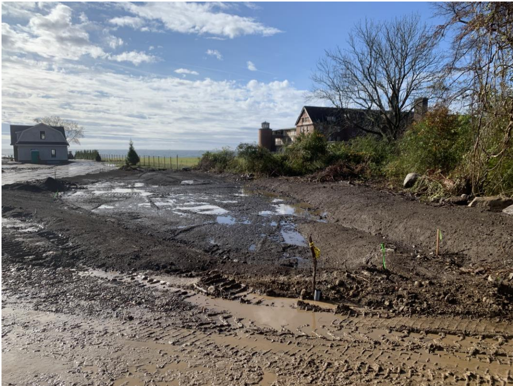
Photo 3: October 15, 2020 – Topsoil Inspection 1:1 Mix of Clean Topsoil & Compost
