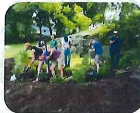
Rain garden installed at Washington Park.
