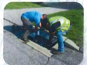
City of Groton Public Works staff install storm drain filter inserts at Groton Estates.
