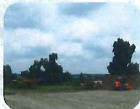
Square A Farm breaks ground on a new free-stall barn for agricultural waste management.
