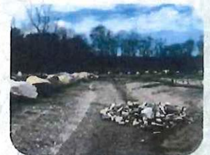
ECCD staff inspect erosion & sediment controls at a solar site in Uncasville.
