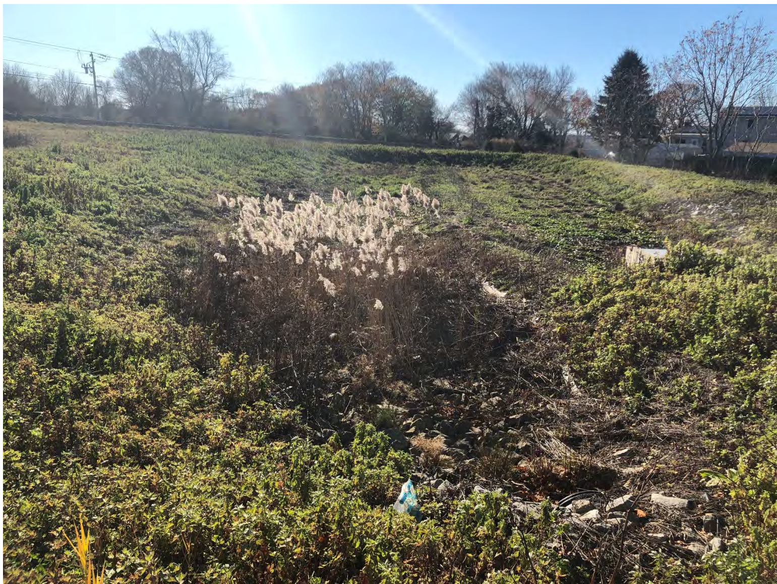
Southern view of southwestern biofilter
