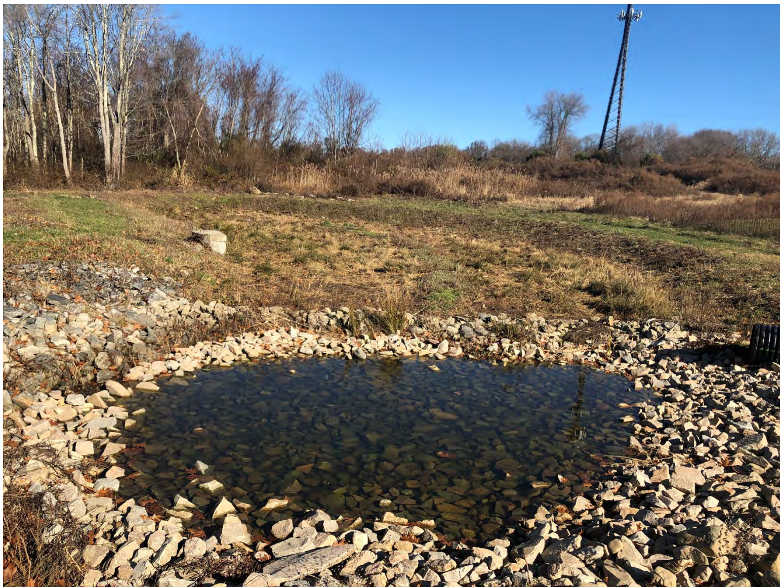
Northern view of northern biofilter
