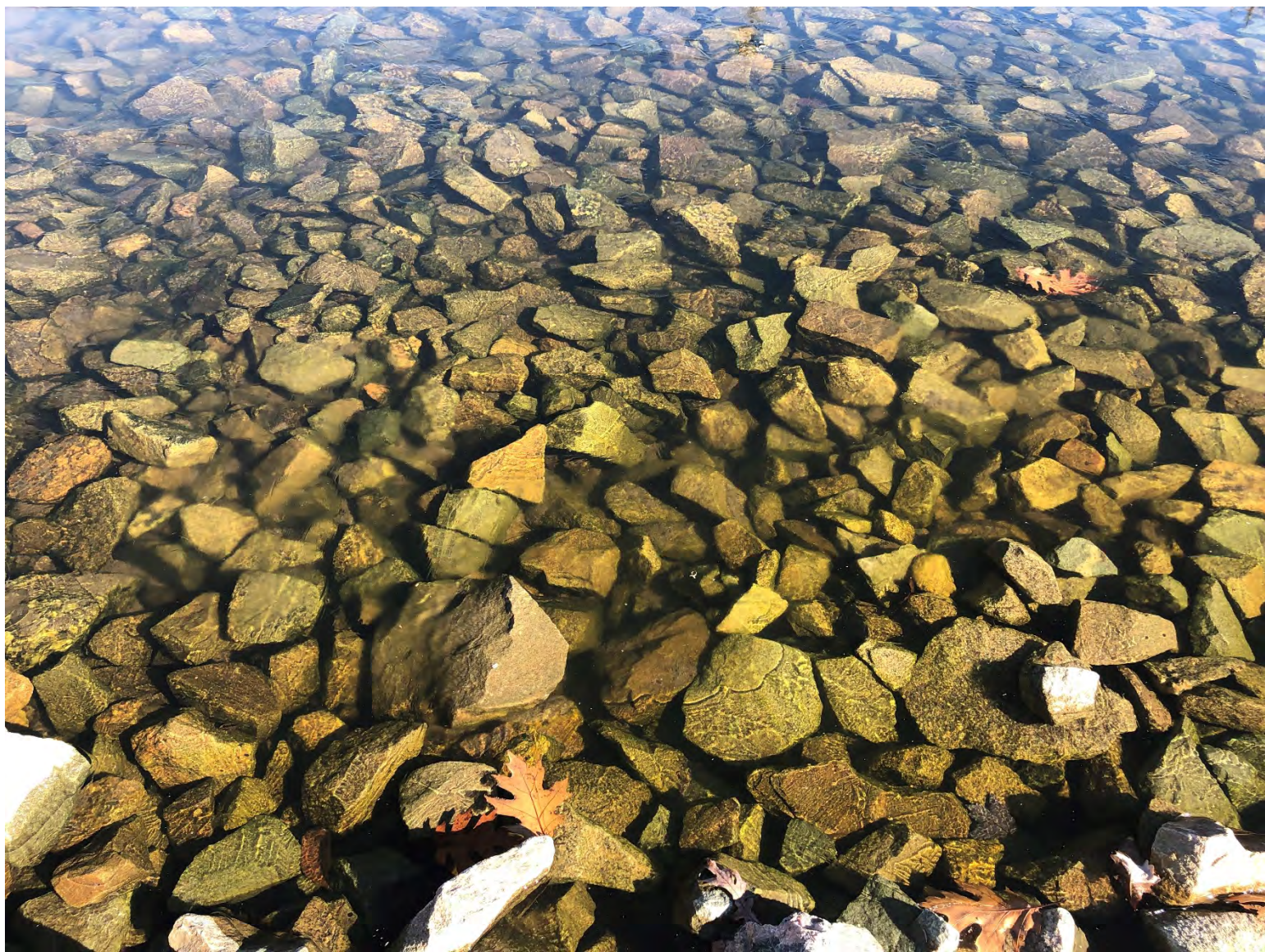
Replaced riprap in northern biofilter forebay
