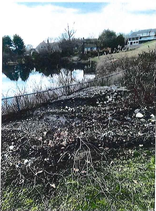
9 Waterview Drive – trench backfill materials eroded to pond 2 1 024
