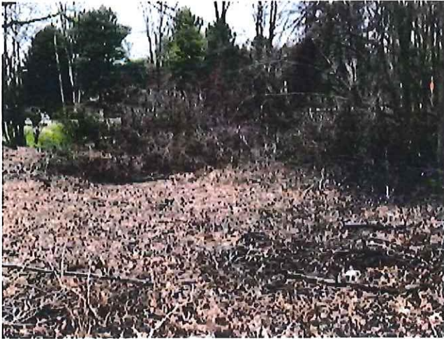
Vines, brush, debris, and briar removal
