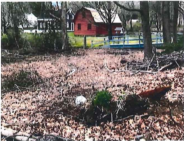
Debris and material to be cleared to allow for better water flow- leaves, branches, etc to be removed
