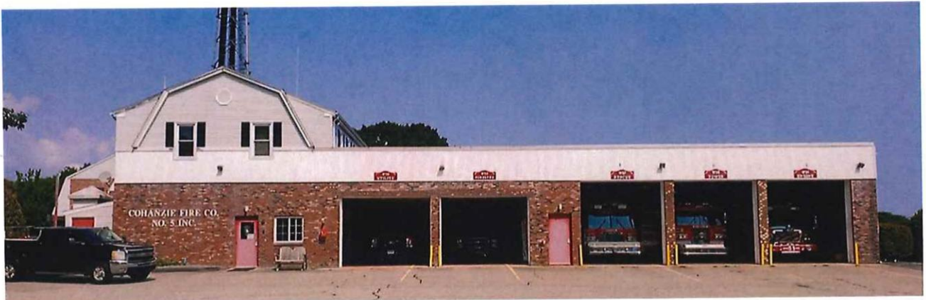
Figure 2- Cohanzie Fire Station
