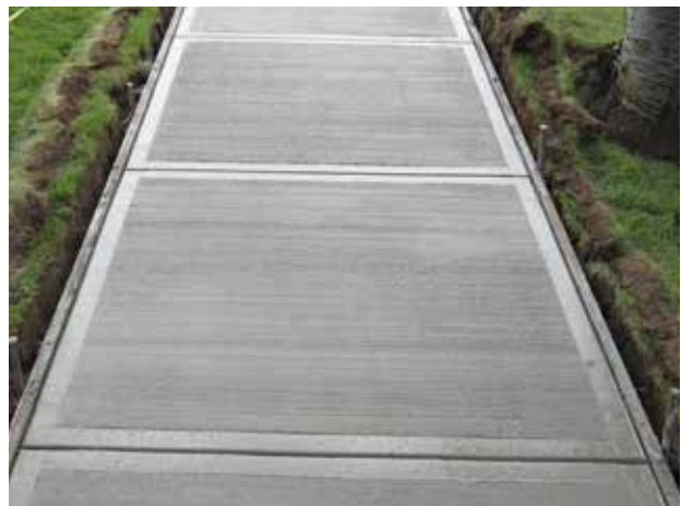
Brushed Concrete Sidewalk
