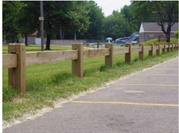
Wood Guard Rail
