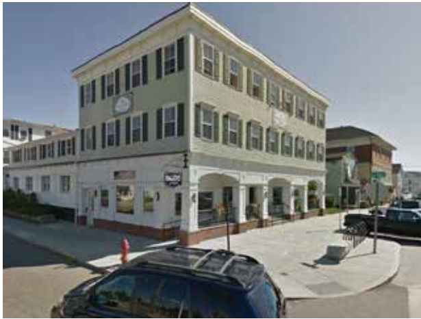
Property Frontage showing Bump-out, Seating and Bike Parking
